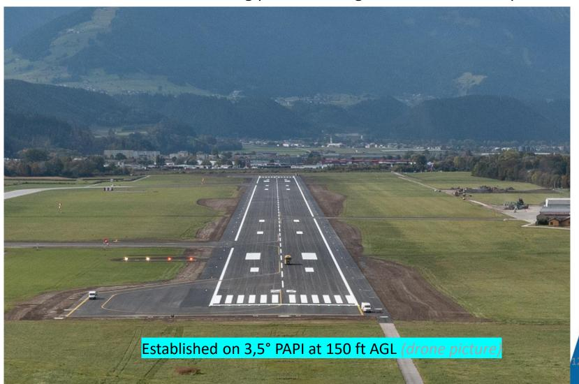
Established on LOC R RWY 26 (LOC/GP-OEV) at DME0,9 at lowest MDA of 2250ft MSL (360ft AGL). BRUCK Same picture as with the old PAPI (3 white, 1 red).
